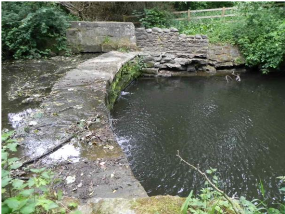
Figure 3 – the concrete cap at the weir crest.
